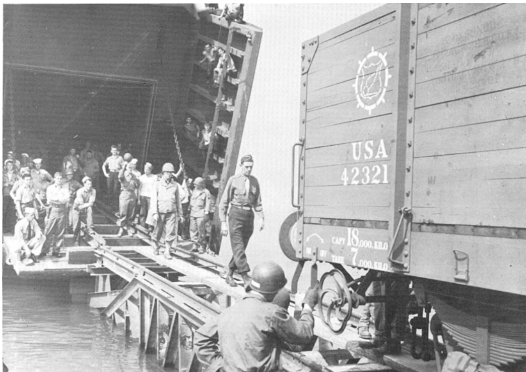
GONDOLA ROLLING OUT OF AN LST, specially equipped to carry rolling stock, Cherbourg, July 1944.
