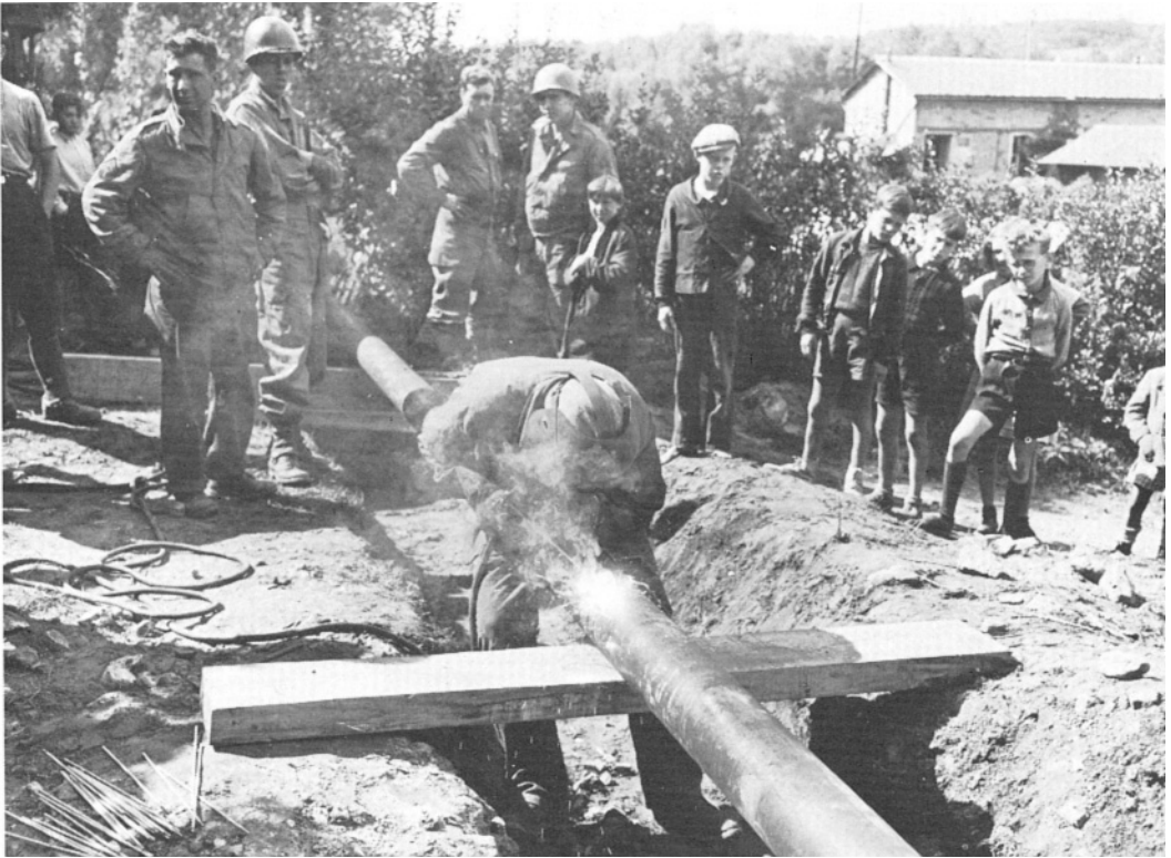
WELDING A SECTION OF THE POL LINE as it is extended eastward across France.
