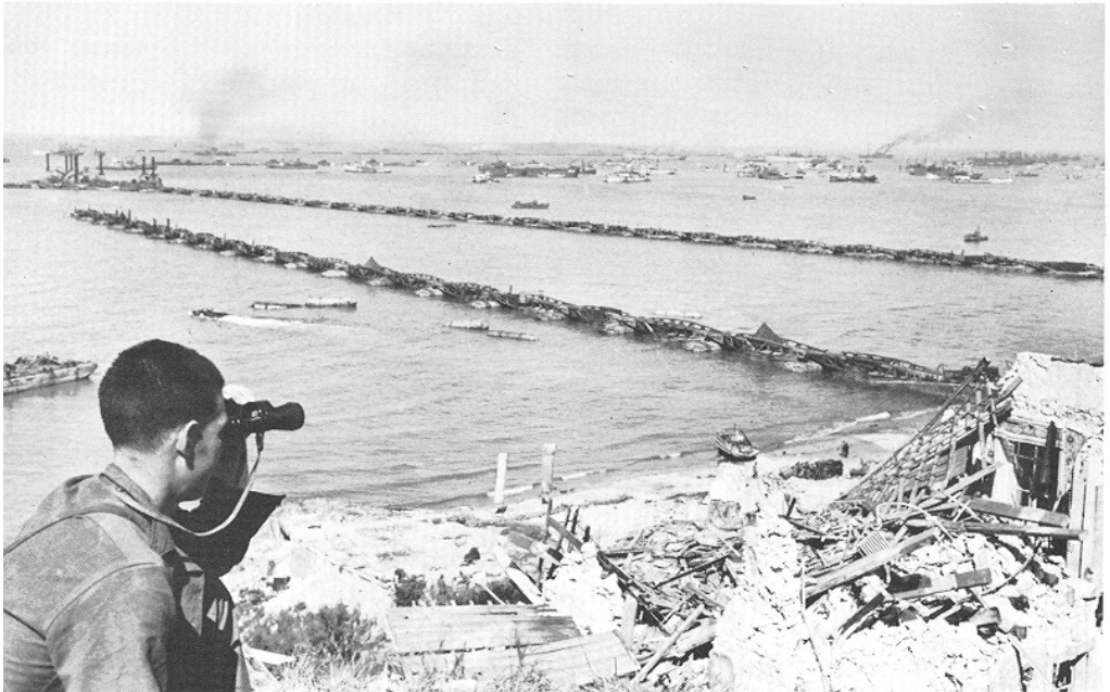
PARTIALLY COMPLETED MULBERRY off OMAHA Beach . Portion of breakwater, above; piers and pierheads, below.
